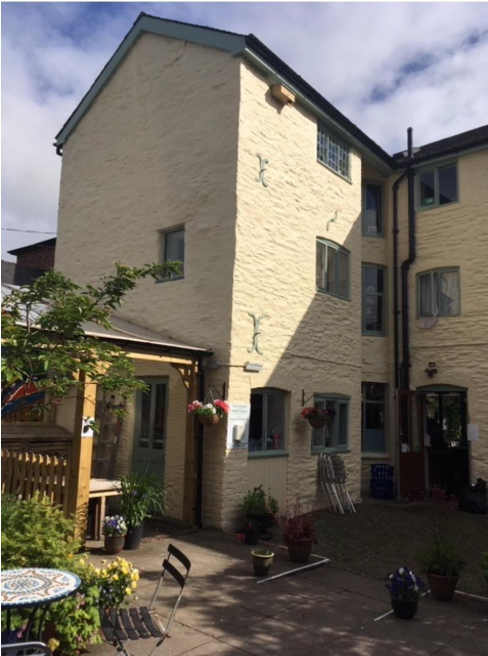
The back of the building showing the new shelter.
